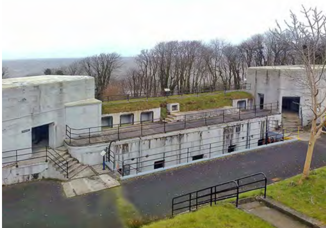
Magazine at Grey Point Fort is between and below the two guns. Photo Conor Stanley
